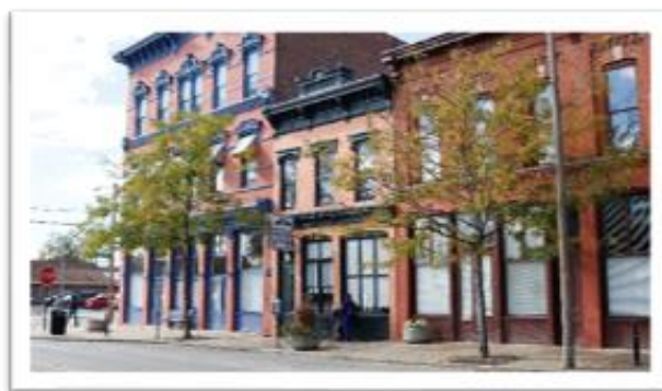
Photo 12: Toledo Warehouse District
